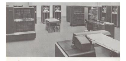
A large-scale data processing system made up of inter-connected units. It can perform up to 42,000 additions or subtractions, or 5,000 multiplications or divisions, each second.
